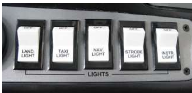
Figure 11. – Lights switches panel
